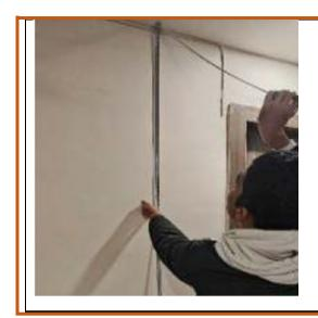
Measuring the wall height from floor to ceiling – **9 feet (108 inches)**
